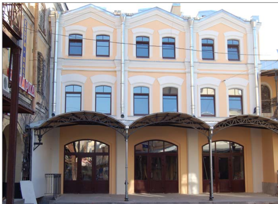
Part of the property development at the Apraksin Dvor 15/16 address, where Ruric carried out extensive reconstruction work during the first quarter 2007
